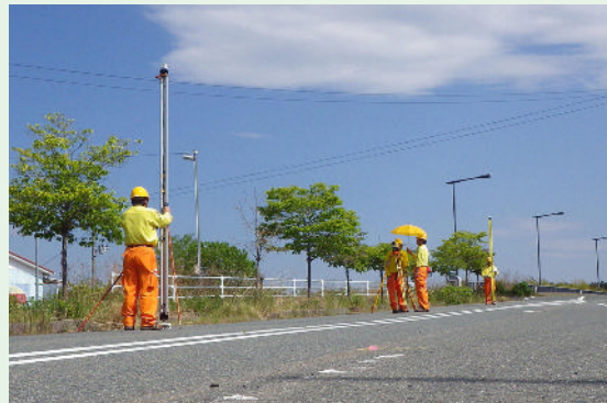
Figure 2 Leveling (performed by a team of four while walking)
