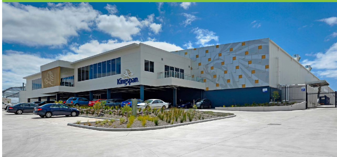
▲ ABOVE/LEFT: Kingspan Insulation Manufacturing Facility, VIC, 6 Star
