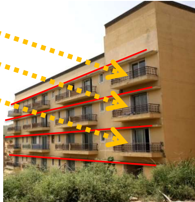
Shading on the south facing windows
