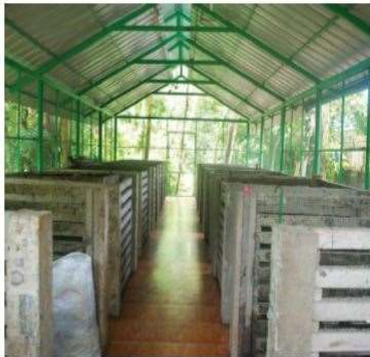
Aerobic Community composting units
