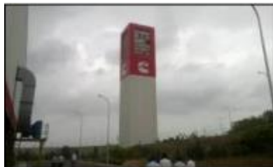
Figure 11: Wind tower of Cummins Generator Technology
