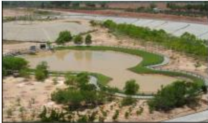
Figure 7: Rain water harvesting pond
