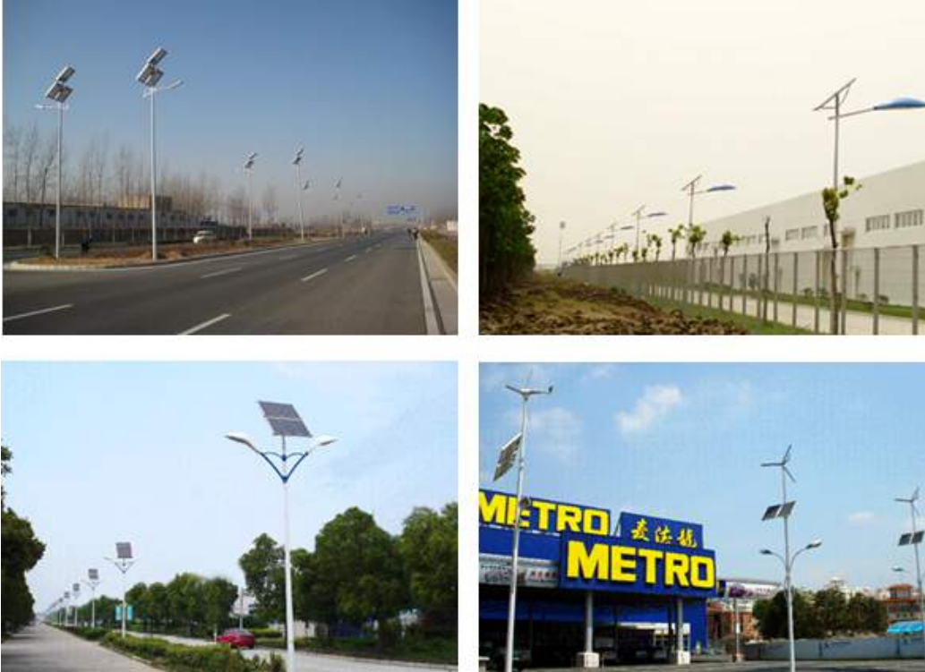
Figure 2- 7: Solar powered public street lighting in low density commercial and industrial areas
