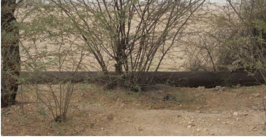
Figure 5- 26: Disused water pipeline running parallel to NH-65 through the Notified Area
