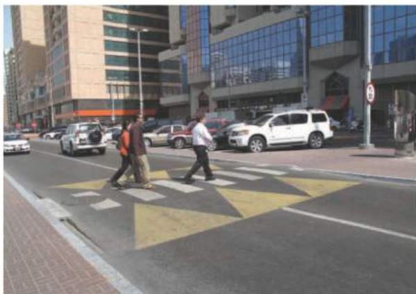
Figure 8- 27: Speed table used as raised crosswalk, Abu Dhabi Source: Abu Dhabi Urban Street Design Manual
