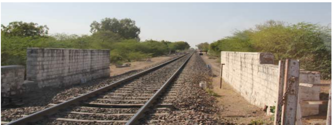
Figure 5- 24: Proposed DFC Feeder Railway line looking north from level crossing junction with SH-64
