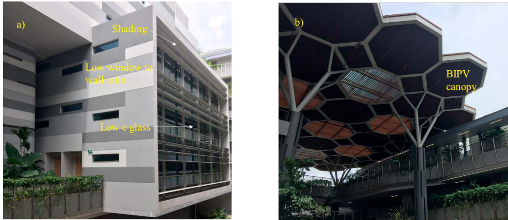
Figure 3: (a) Contributing factors to low ETTV (b) Building Integrated Photo-Voltaics (BIPV) canopy
