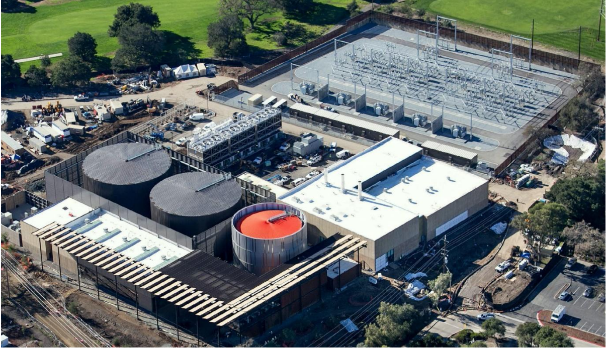
Figure 5.1 Stanford University energy supply
