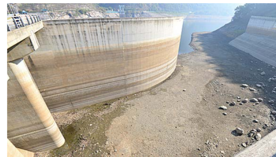
Figure 15. Water gate of Boryeong revealing its bottom (2015.10.24) (Source: K-water)
