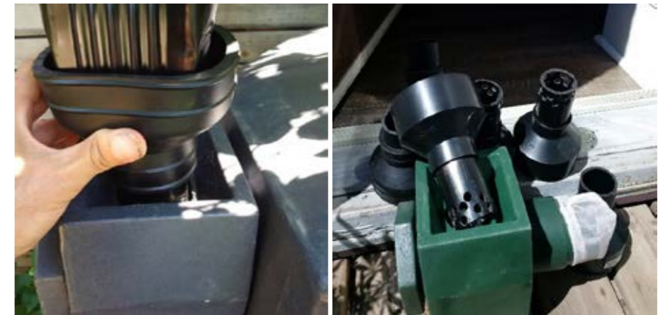
Figure 13. Riverside Storm funnel in diverter box (left); uninstalled storm funnels (black) and diverter box (green) with filter (white)
