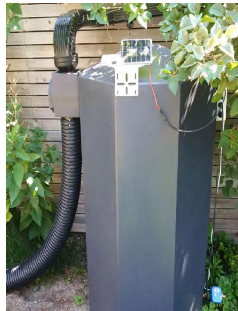
Figure 11. Installation of RSSUT system in the Riverdale pilot (Source: Riversides)
