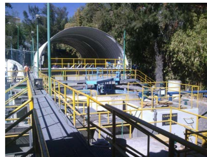
Figure 10. "Cerro del Agua", main Wastewater treatment plant of the University City, in 2008. It comprised: a) Pre treatment: sand traps and screens for elimination of large solid particles; b) Flow meters: three flow meters parallel to each other; c) Secondary treatment: Activated sludge treatment, rotatory biological discs, and spray filter (all used within the same WWTP); d) Tertiary treatment: sand traps (filters) and disinfection. (PUMAGUA 2012)
