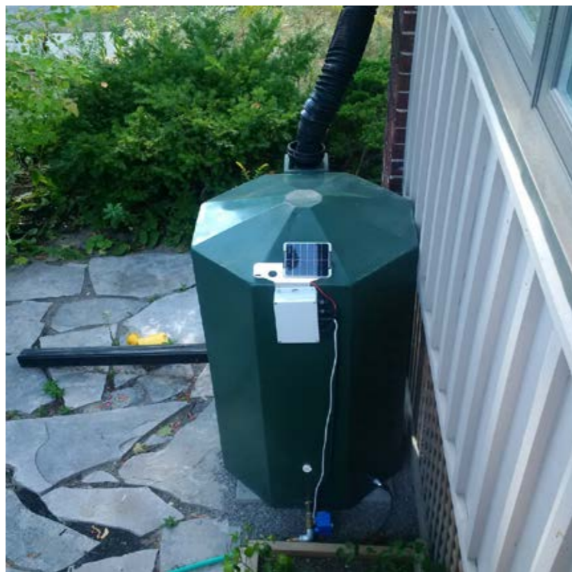
Figure 8. Stormwater Smartgrid cistern
