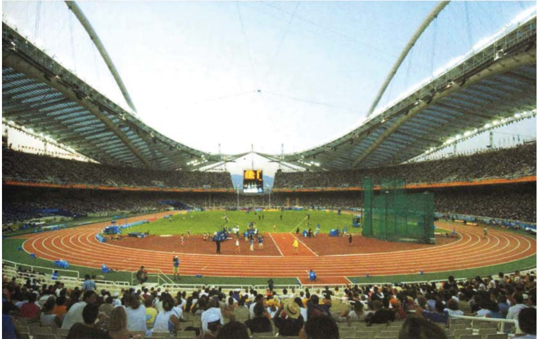
Illustration 36: Athens Olympic Stadium with a capacity of 72,000 seats and new roof structure during the Olympic Games in 2004 268
