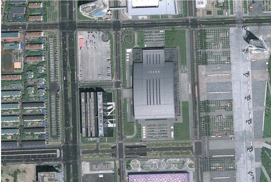
Illustration 48: Satellite picture of Beijing Indoor Stadium (centre) and precinct with swimming stadium below 291
