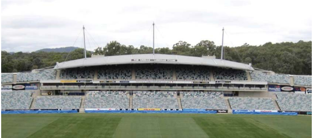
Illustration 31: Canberra Football Stadium with roof above the grand stand with 8,000 covered seats constructed for the Olympic Games in 2000 257
