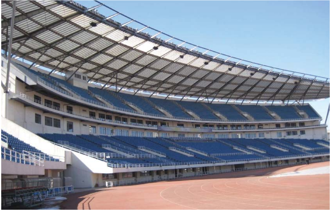
Illustration 53: Beijing Football Stadium with new roof structure (permanent overlay) after the Olympic Games in 2008 297
