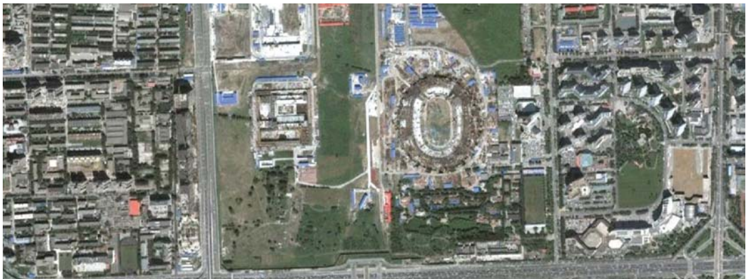
Illustration 55: Satellite picture of Beijing Olympic Stadium dated 18.08.2005 during construction works for the Beijing Olympic Stadium and Olympic Park 302
