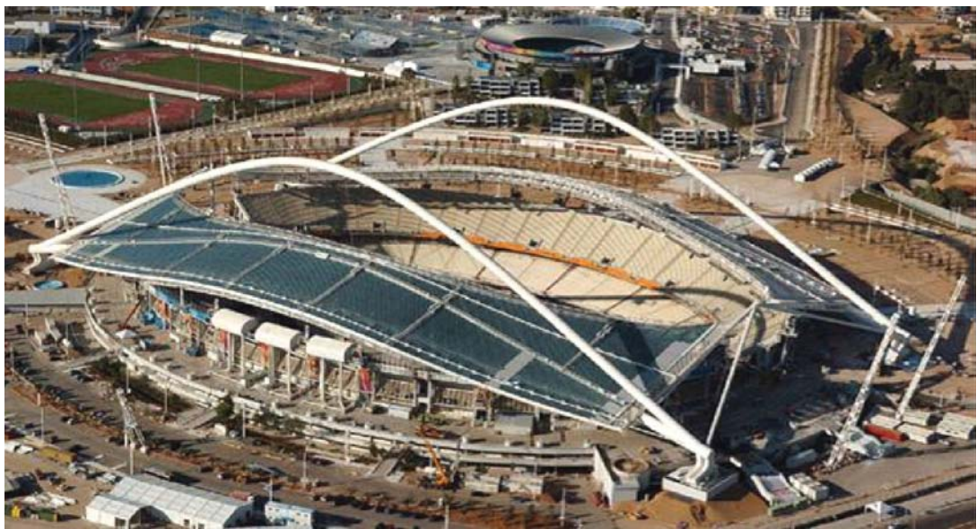
Illustration 35: Athens Olympic Stadium with spectator capacity of 71,030 seats during construction 267
