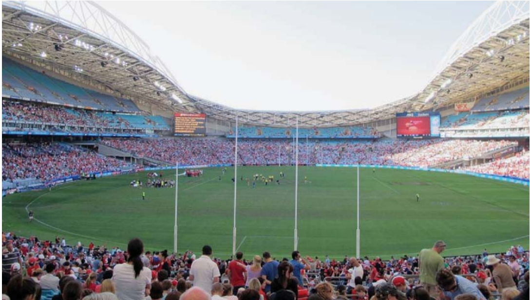
Illustration 25: Sydney Olympic Stadium with reduced seating capacity of 80,000 after Olympic Games and new roofs above modified north and south spectator stands 241
