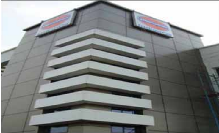
Figure 15.2: IOCL DO Office Building, Indore
