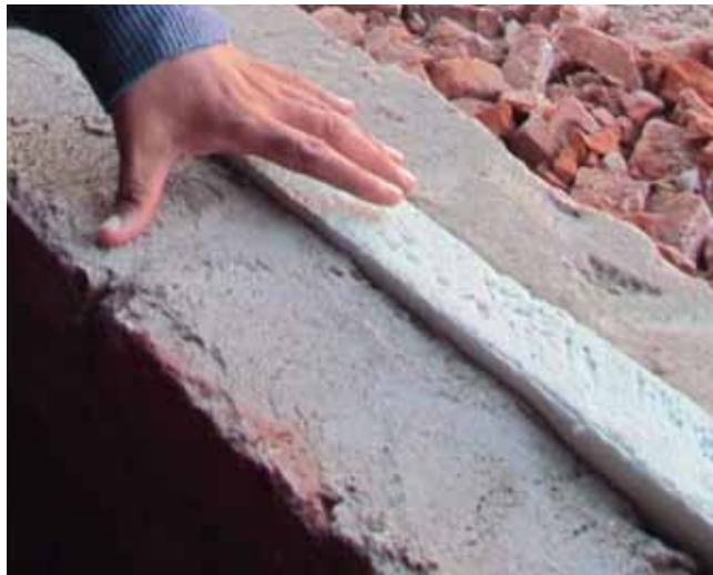
Figure 16.5: Cavity wall insulation
