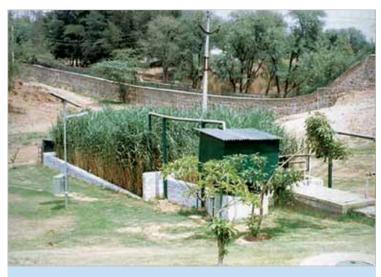
Figure 7 Root zone system for waste water treatment
