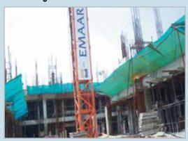
Figure 4 Safety nets at construction site
