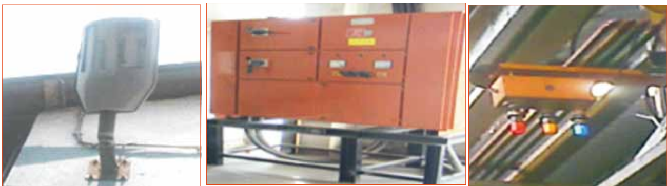
Figure 1: Some Initiatives (Left to Right) Magnetic Induction Lamp, Voltage Control and 15 W indicator bulbs
