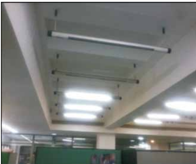
T5/CFL (Before) replaced with LED Lighting (After)
