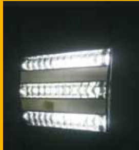
Before with 3X36Watts CFL light fixture
