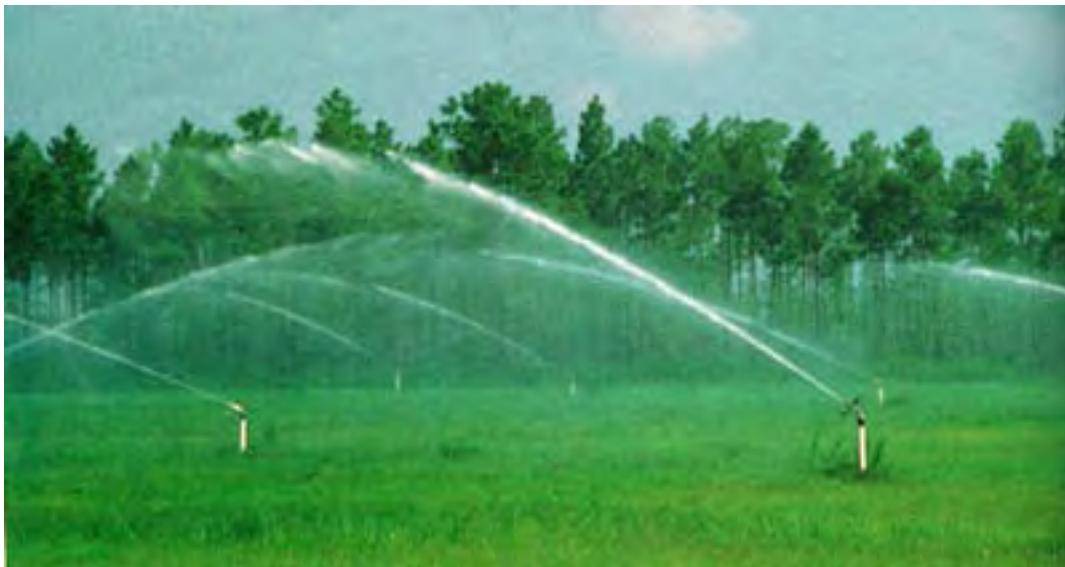
Spray irrigation is used for effluent treatment and disposal at West Jackson County during dry weather.
