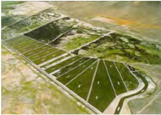
Wetland treatment cells with islands were constructed around the existing warm-water wetlands.
