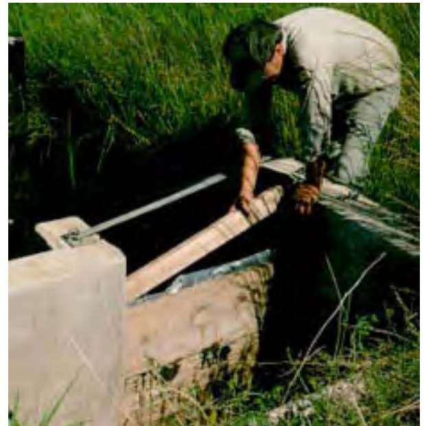
Water control structure at Redhead Marsh.
