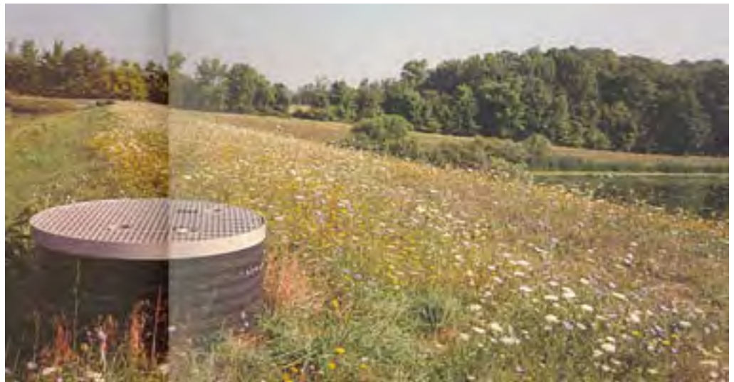
The ponds at Vermontville are set into a hillside that drops off more than 70 feet. This view of lagoon 2 shows the high and wide berms that this relief necessitates. In late summer, these are covered with a profusion of wildflowers.
