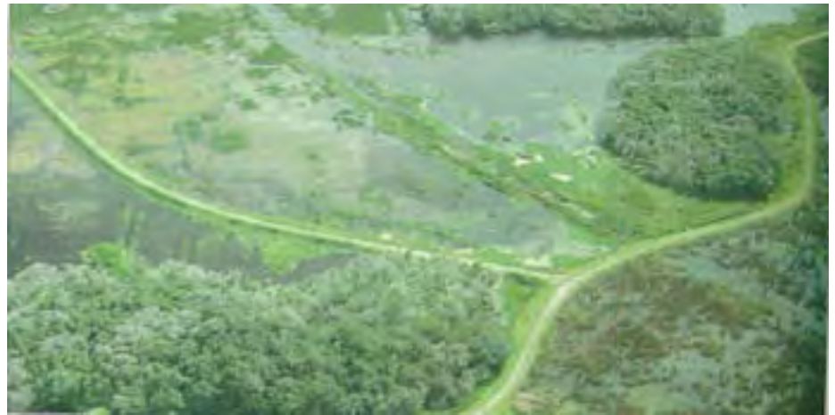
Berms divide the 1,220-acre wetland system into treatment cells which provide additional nutrient removal to treated effluent passing through the site.
