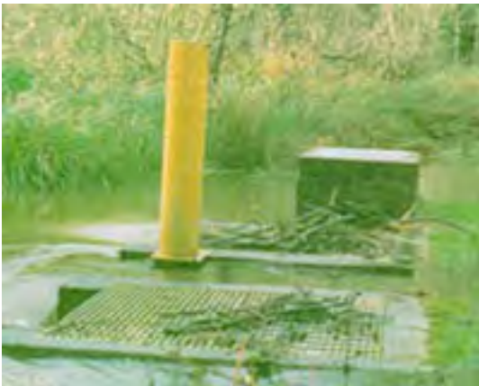
Effluent structures during winter flooding (when wetlands are typically not operated).
