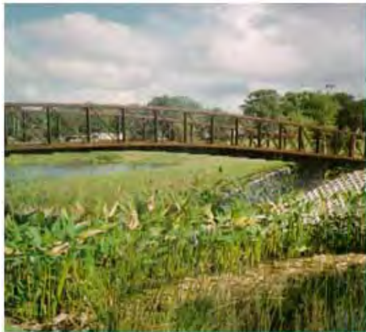
Constructed wetlands are being effectively used to help protect the quality of urban lakes by improving the quality of stormwater runoff in urban areas such as at the Greenwood Urban Wetland, a former dump site, in Orlando, Florida.
