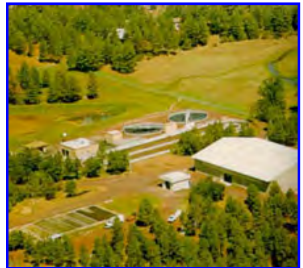
Aerial view of treatment facility.
