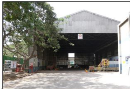
Covered Storage Area
