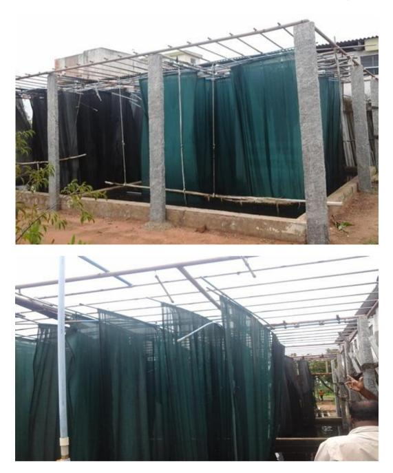
**Figure 2:** Photo plate of Net Evaporator for ZLD of Spend Dye bath at M/S Suntex Processing Mills, Chennai for 40 cum / day of wastewater at about 55,000 mg/L of TDS
