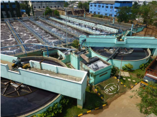
Figure 11. Pallavaram CETP/ZLD, Aeration and clarifier tanks; Ultrafiltration units; Reverse osmosis; Multiple evaporators
