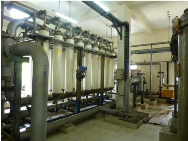
Figure 11. Pallavaram CETP/ZLD, Aeration and clarifier tanks; Ultrafiltration units; Reverse osmosis; Multiple evaporators
