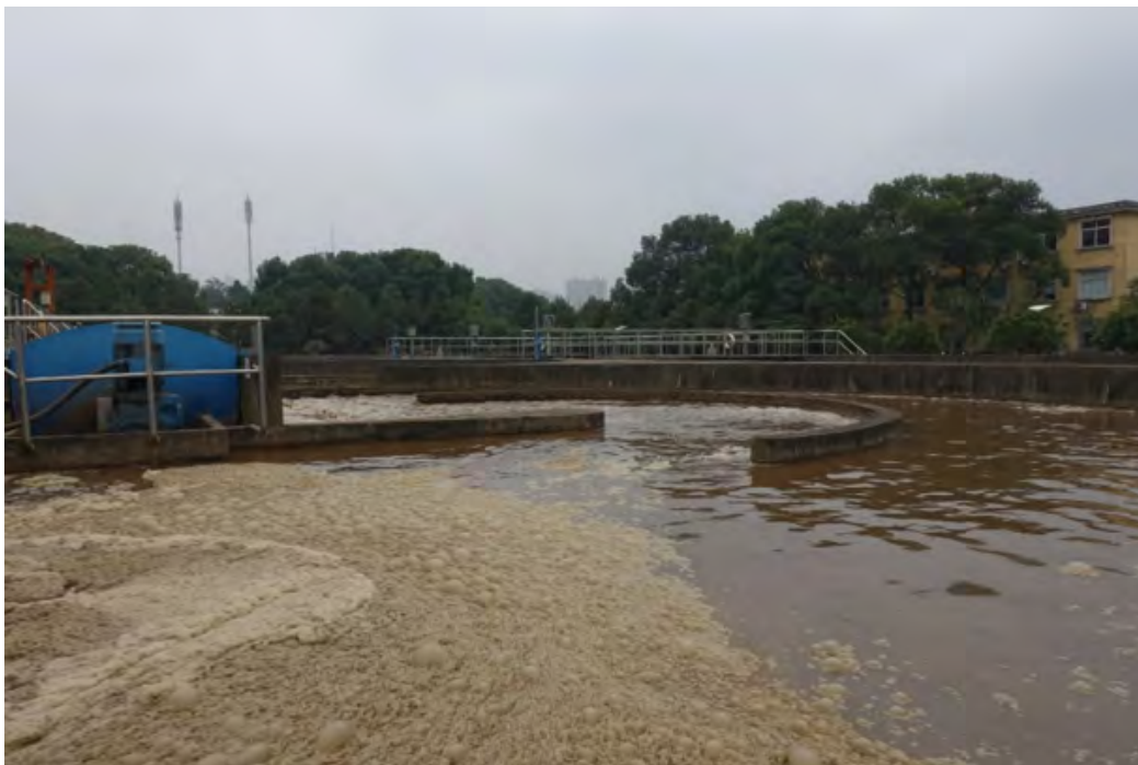
Figure 32: Photo of an oxidation ditch, China
