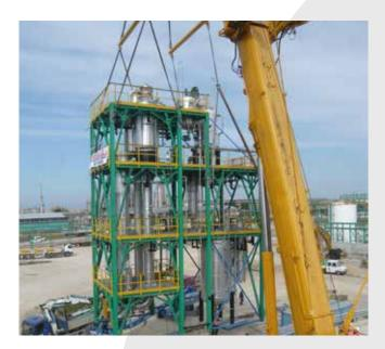
For small-scale applications, a skid-mounted modular concept has been developed to recover high quality process condensates and separated (disposable) solids, meeting the critical reliability and availability requirements of a power plant.
