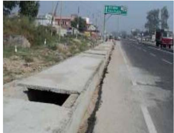
Figure14: Drain on Left Side at Km 74.840
