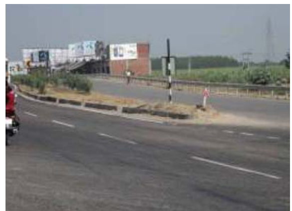
Figure 22: Minor Junction at Km 86.750 Storage lane not provided
