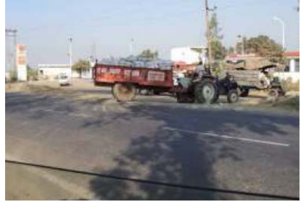
Figure 24: Unauthorized Median Cut at Km 113.210: Unauthorized Median cut should be closed wherever possible. Temporarily proper sign board should be installed.
