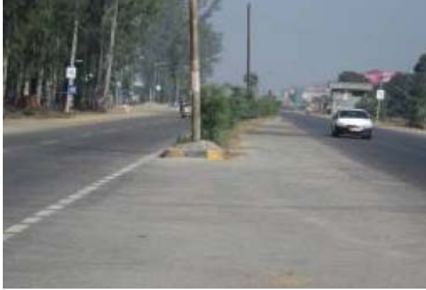
Figure 17: Median Opening at Km 77.835 • Object Marker not provided. • Pavement Marking missing.
