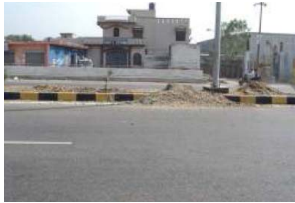
Figure 18: Underpass at Km78.350 Soil should be removed from the carriageway
