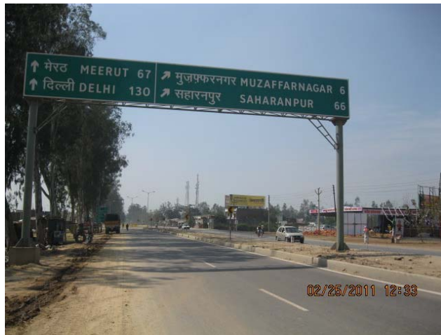
Figure 4: Divided Four Lane at Km 130.00 (Muzaffarnagar By-pass) on NH-58 in Opposite Direction
