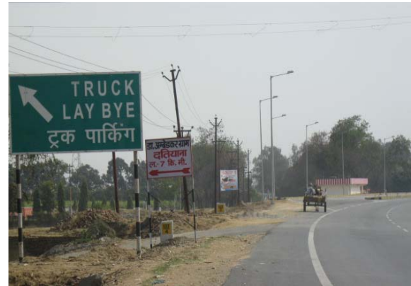
Figure 26:Confusing information board of Truck lay bay at Km 122.400
