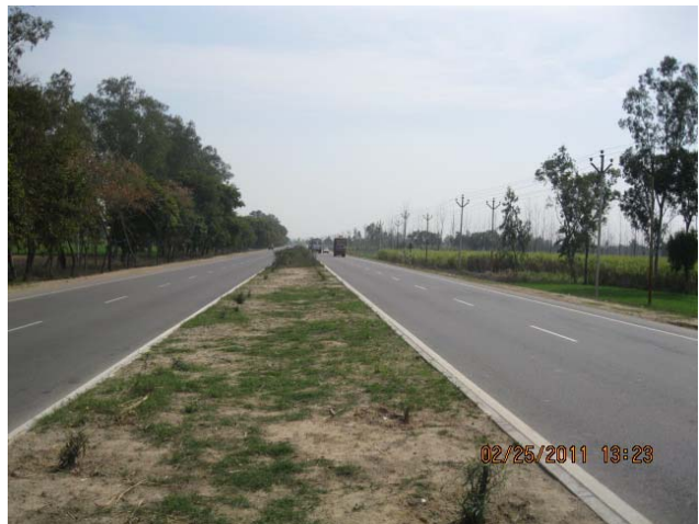
Figure 5: A View of a Section of Four Lane National Highway-58
