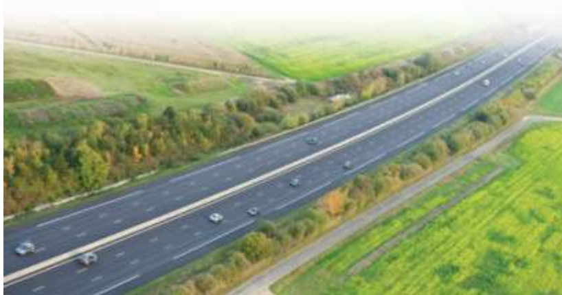
Natural Disaster may affect Expressway evacuation management due to limited assess
