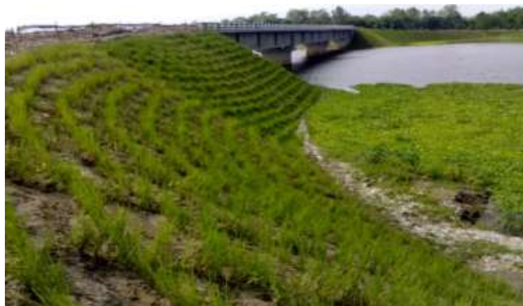
Vetiver Grass used for Slope Stabilization in Bridge ↑ & Road ↓ Embankment
