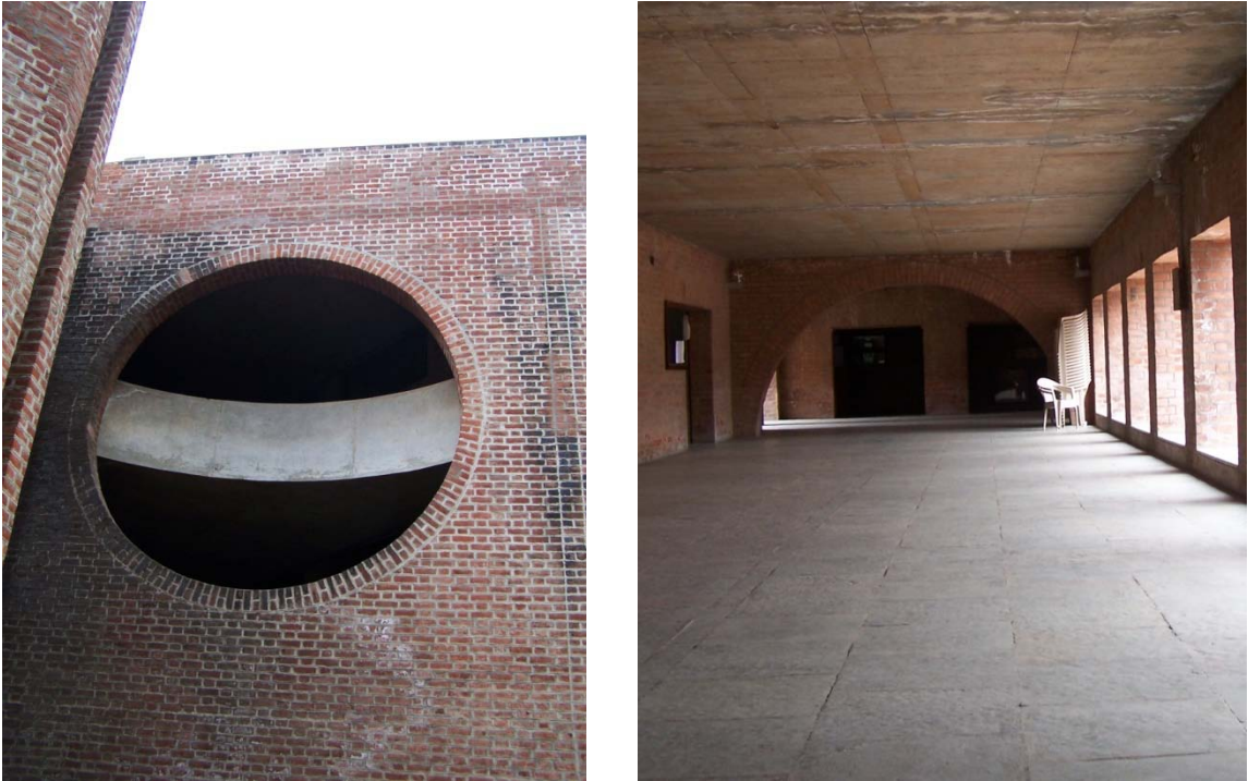
Figure 2.18 and 2.19: Use of brick and concrete façade integrated with light wells and deep corridors to create spaces with natural light and natural ventilation: IIM Ahmadabad, Louis I. Kahn
