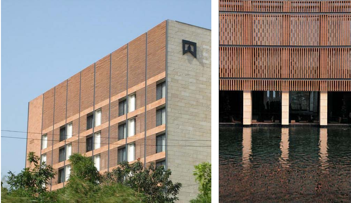
Figure 2.26: Use of modern building materials following traditional screening system on façade – ITC Sonar Bangla Hotel; Kolkata, Kerry Hill. Figure 2.27: Detail of facade
