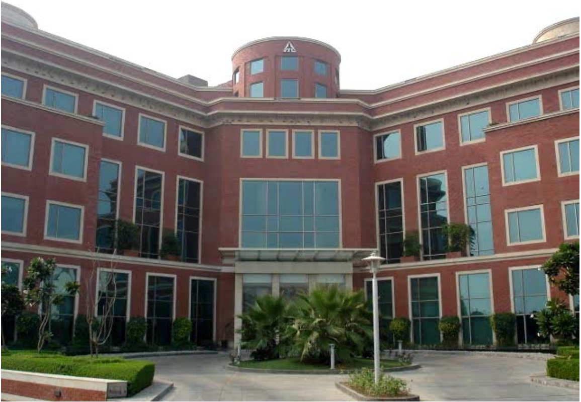
Figure 1.2: ITC Green Center, Gurgaon, India, 2005, LEED New Construction Platinum rating: Insulated glazing is used to minimize solar heat gain, External air economizer draws fresh air in mechanically, but the building skin lacks additional external shading elements to counter the high solar angle and depends entirely on a mechanical HVAC system without any provision for natural ventilation. Image Courtesy: Neha Gupta
