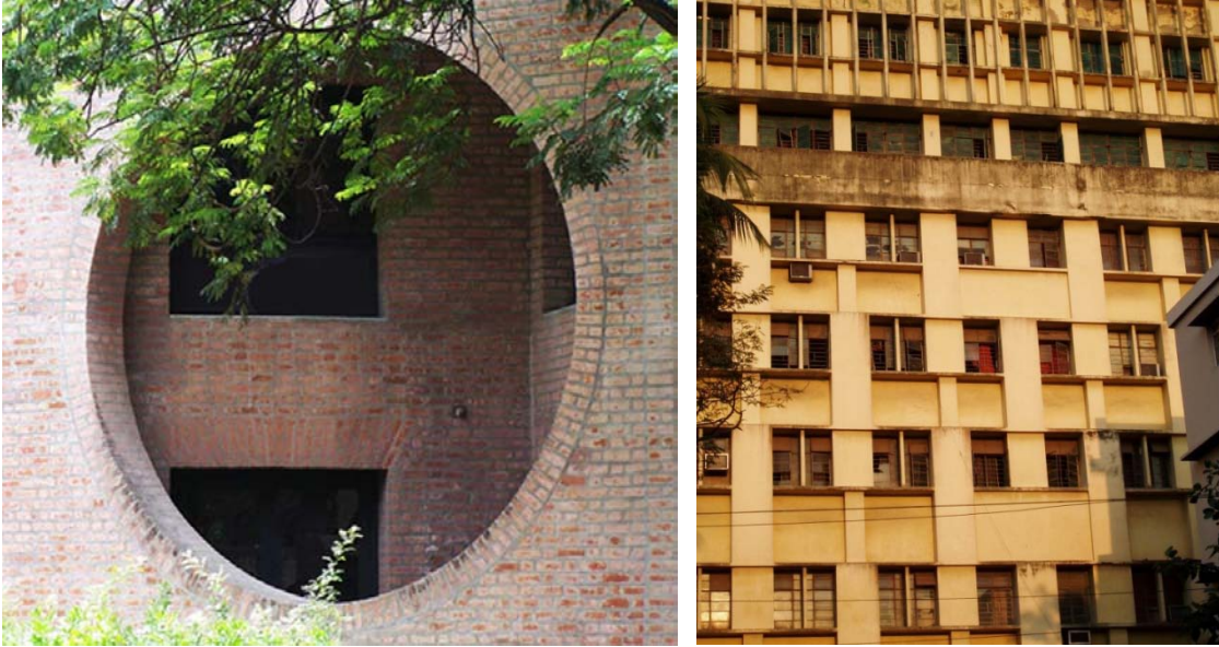
Figure 2.9: Openings to allow airflow while preventing direct exposure from sun: IIM Ahmadabad, Hot-Dry climate
