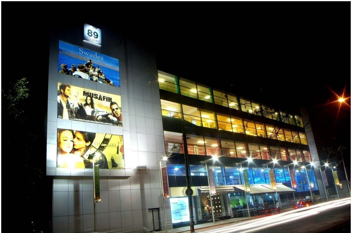
Figure 2.25: Extensive use of aluminum cladding and glazing with little consideration for the heat and ventilation: Cinema 89, Kolkata. Image Source: Bengal Ambuja Pvt. Ltd.
