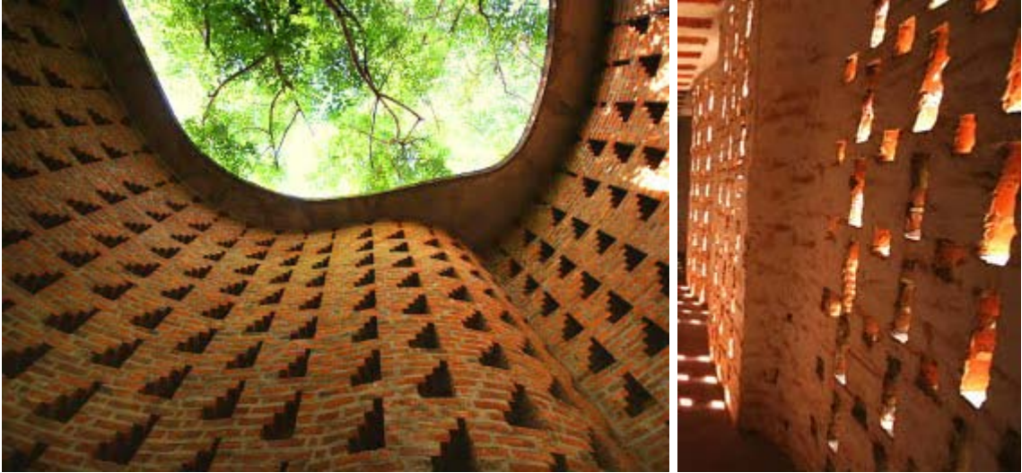
Figure 2.21 and 2.22: Use of small openings to allow daylight and air while blocking the heat, an example of synergy of techniques: The Centre for Development Studies, Trivandrum; Kerala, Laurie Baker. Image Source: www.laribaker.net
