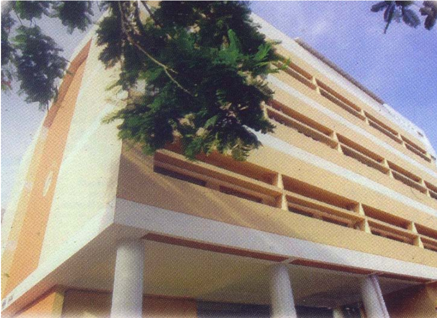
Figure 3.17: WEBREDA Building, Kolkata, India
