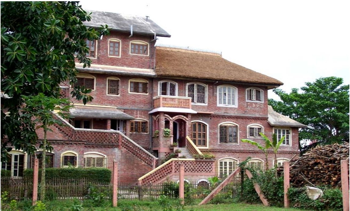
Figure 2.20: Combination of brick walls, concrete and thatched roof, and window projections to provide solar protection: ISCON Housing; West Bengal, Laurie Baker
