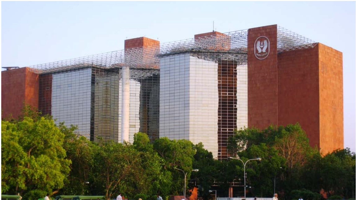
Figure 2.24: Combination of traditional stone and modern glazing in façade with solar protection added by overhead space frame acting as shading device – LIC Building, New Delhi; Charles Correa
