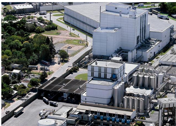
Mastellone Hnos, the biggest dairy company in Argentina. General Rodríguez Industrial Complex.
