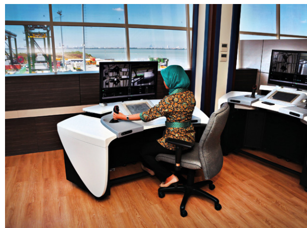
Fig. 3: Supervision of operation of the ASC is performed from a remote office
