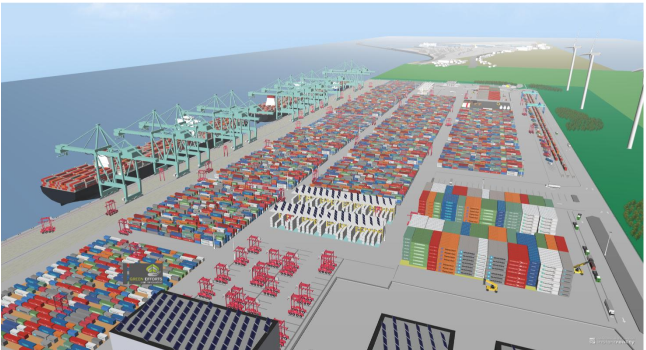
Container terminal and Trelleborg RoRo terminal overview
