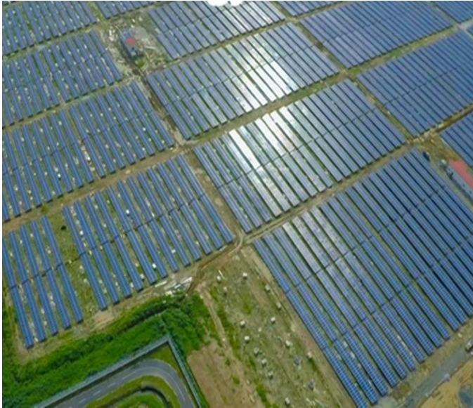
PICTURE 10: Image of solar panels in Cochin Airport
