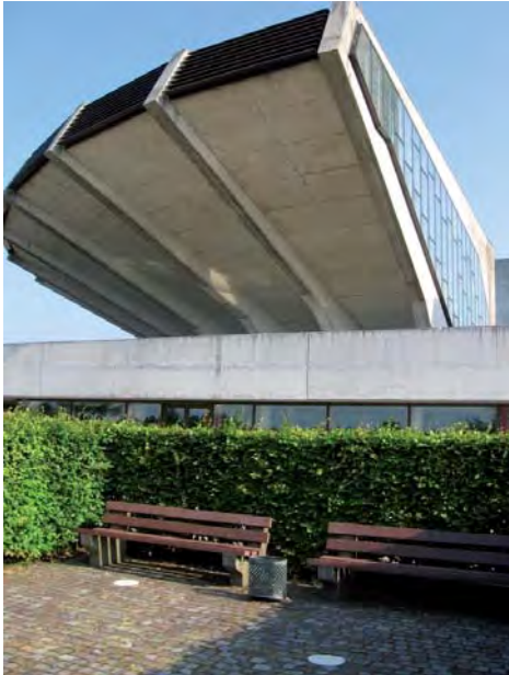
Photo 14 The high hedges conceal the GOE at Herlev Hospital from being seen from inside the building.
