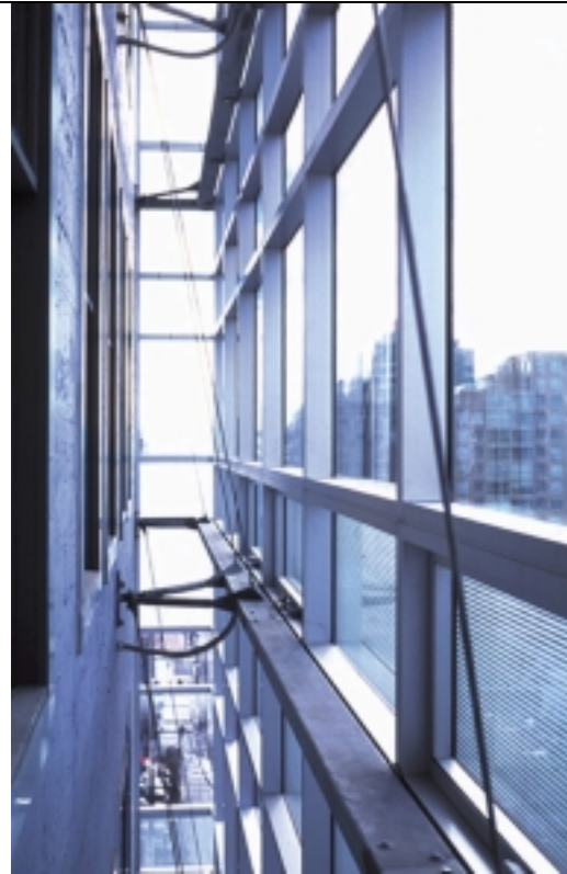
The Telus Office Building, above, uses 30% Less Energy Than ASHRAE 90.1. The third skin creates an air gap which keeps heat in during the winter and provides shade in the summer. Reprinted with permission by Busby + Associates.
