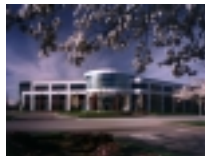
Crestwood Centre courtesy of Bunting Coady Architects
