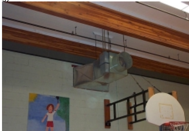
The solarwall system in place at Charlie Lake School gymnasium, Peace River School District #60, Fort Saint John, BC. Photograph above, solarwall on building exterior; photograph below, interior detail in gym.
