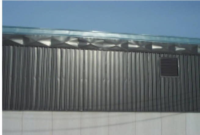
The solarwall system in place at Charlie Lake School gymnasium, Peace River School District #60, Fort Saint John, BC. Photograph above, solarwall on building exterior; photograph below, interior detail in gym.
