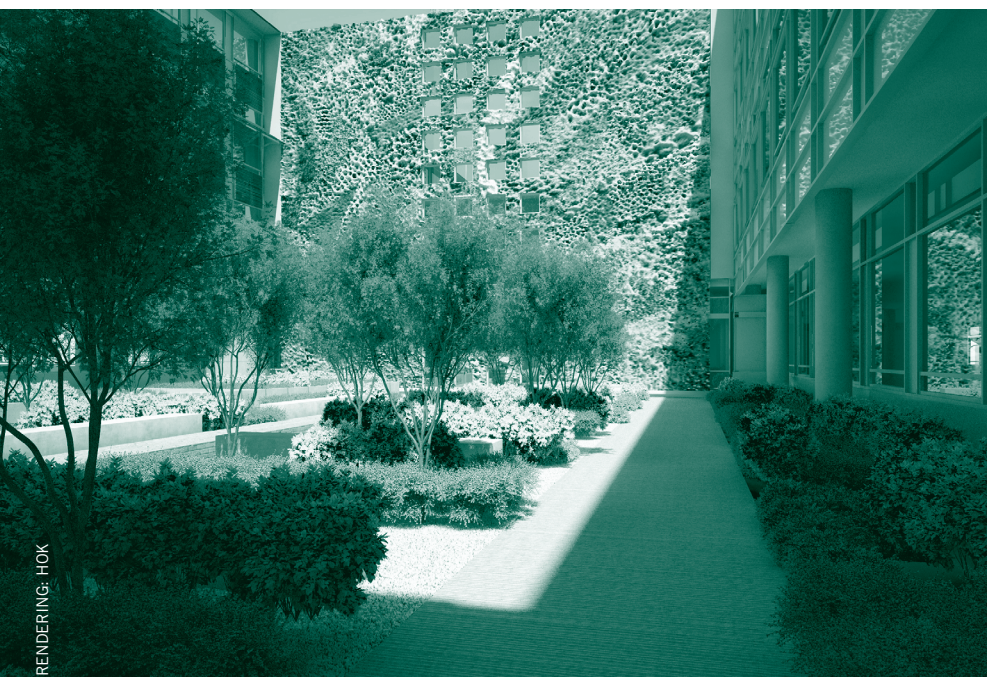
Water wall garden in the net-zero carbon office prototype. Vegetated walls along the east and west facades of the links between the office bars provide aesthetic continuity and moderate the outdoor climate. The south facade has an edible food garden area (not shown) as an additional amenity for building occupants.
