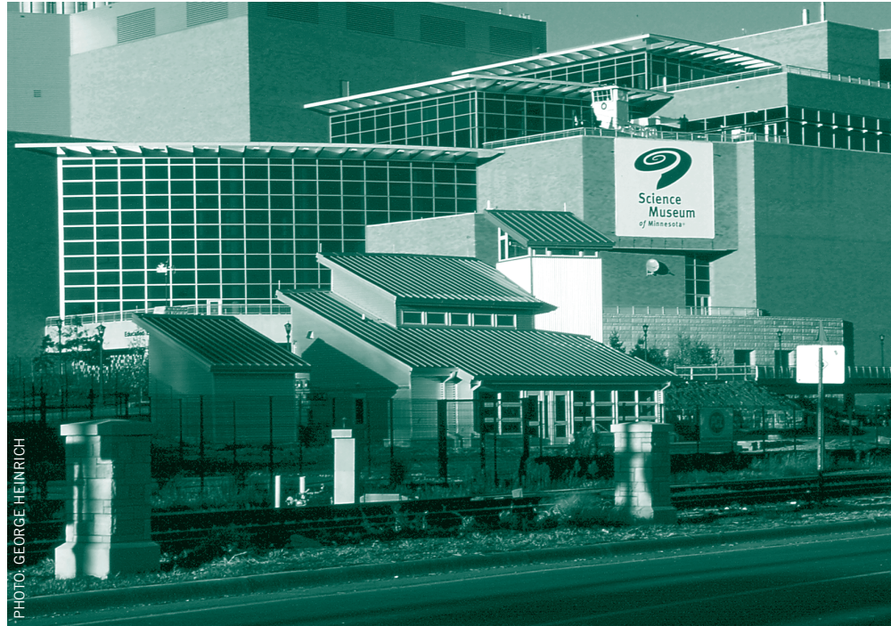
The 1,700-sf Science House (at center in photo) features an 8.8 kW photovoltaic array and ground-source heat pumps. The Building Team consisted of Barbour LaDouceur Design Group (architect), Vareberg Engineering (EE), Martin Mechanical Design (ME), The Weidt Group (environmental consultant), and LS Black Constructors.
