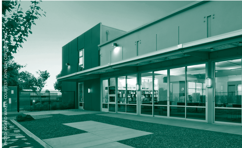
The Z 2 —for “net-zero energy, net-zero emissions”—IDEAs office building in San Jose, Calif., uses high-efficiency electrochromic windows and skylights to take advantage of daylight and operable windows to permit natural ventilation. Photovoltaic panels, part of the single-ply roof, provide the facility’s energy source. A Johnson Controls Metasys building management system controls the geothermal heat pump and radiant floor system.
