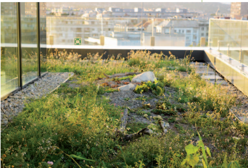
Biodiverse Green Roof in Hungary, Budapest: a mix between extensive and intensive structures addressing pollinators needs (Dezsényi, Malmberg, Enzi 2013)
