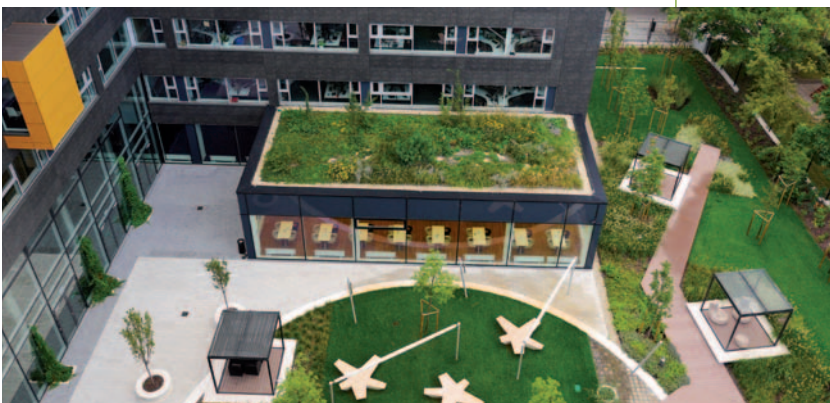
5 different Green Roofs and Walls on/in LEED Platinum certified Green House Budapest (Dezsényi, Malmberg, Enzi 2014)
