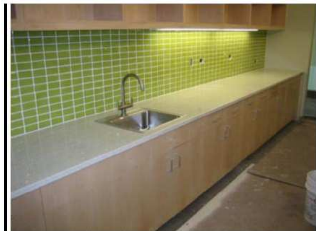
Countertops and backsplashes are made from recycled glass.
