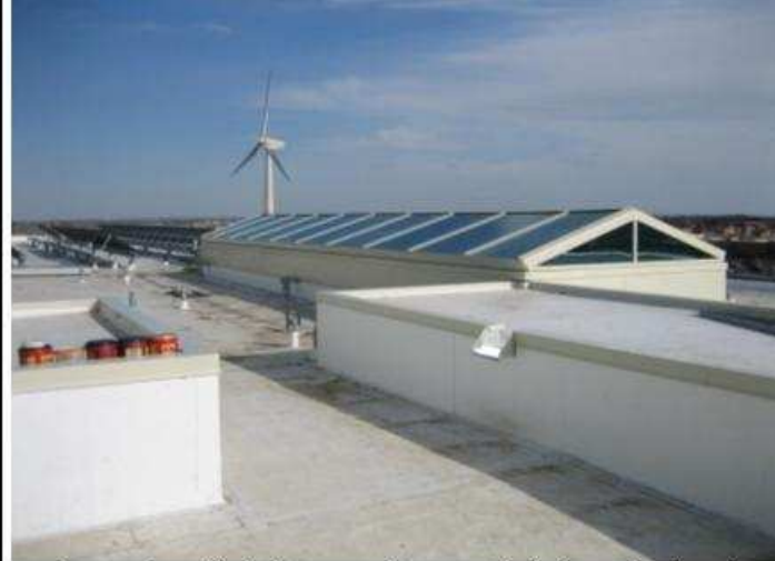
A white roof and daylight atrium harvest daylight and reduce the energy needed for lighting.
