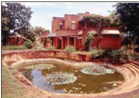
Biological wastewater treatment
