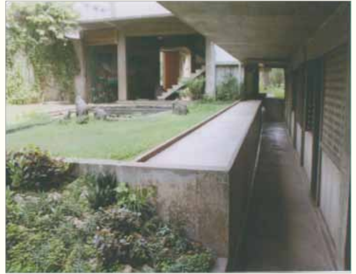
View of entrance from the basement
