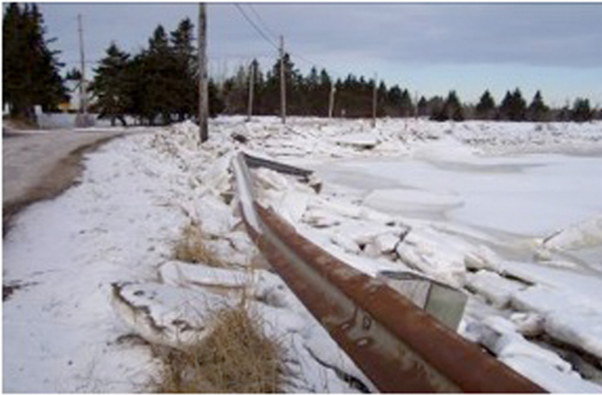
Winter storm surge damage - TPDC staff photo
