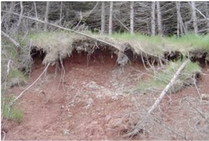
Ongoing coastal erosion - TPDC staff photo
