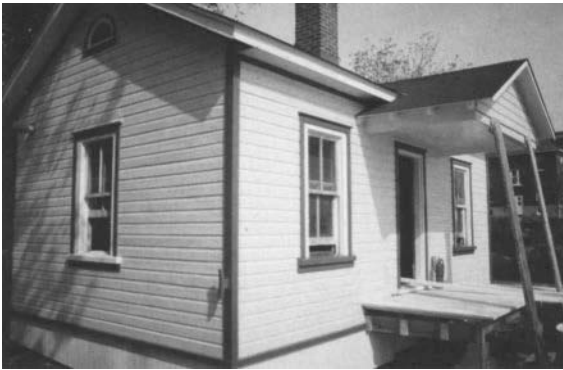
The Marconi Station in September 2001. Built in 1919, the Marconi Station is a small building with a double-sided roof. It is set back from the road, close to the river, and not far from the physicians' residence. The utilitarian role of the building is reflected in its interior arrangement: the console and its operator were in the western half, and the generator and washroom were in the eastern half. The Marconi Station replaced the old telegraph office between 1885 and 1892. The building demonstrated the technological advance in communications as well as the daily operations of a human quarantine station such as Gross Île.
