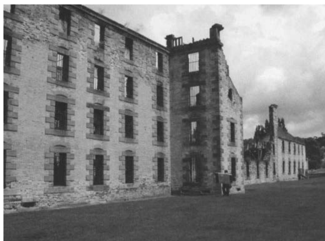
Figure 3.6. The penitentiary building, the largest and most prominent structure from the convict period. Photo: Marta de la Torre
