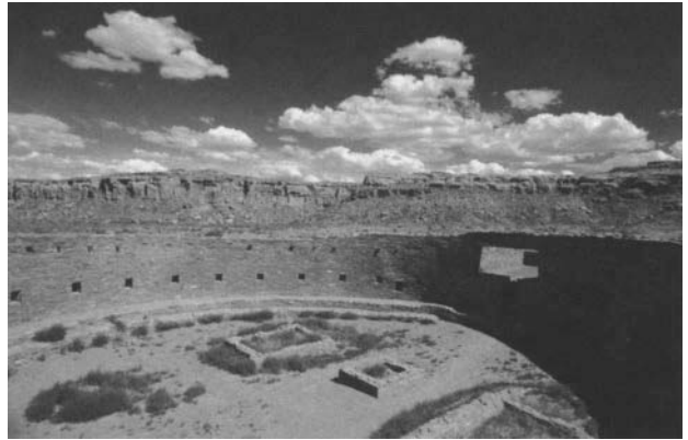
Casa Rinconada viewed from above. For several years during the time that Casa Rinconada—the largest kiva in the Park—was open to visitors, a shallow layer of dirt protected the floor features. Recently, the features were uncovered after access to the interior was prohibited. Both Native American sensitivities and conservation concerns influenced this decision. Photo: Guillermo Aldana
