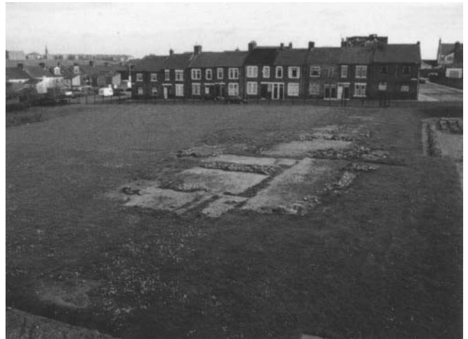
Figure 4.5. The exposed foundations of a fort at South Shields. Photo: Margaret G. H. MacLean
