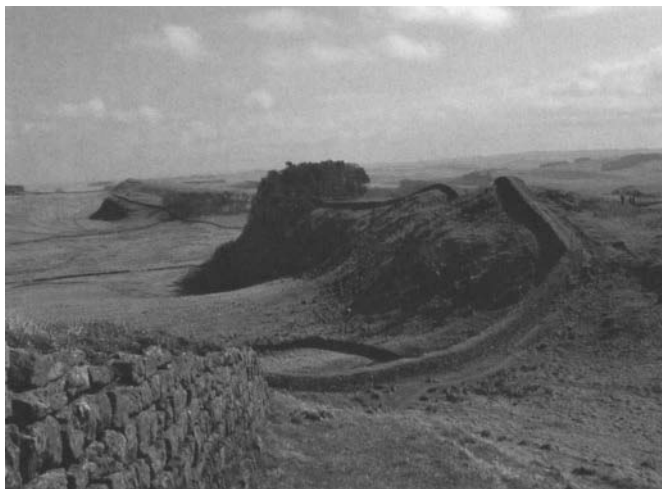
Figure 4.8. The Romans took advantage of the landscape's natural barriers, situating the Wall atop the high ridges of Whin Sill, east of Housesteads. Photo: Marta de la Torre.
