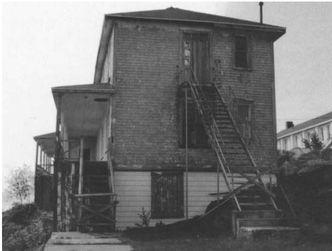
Figure 1.13. Now called the Second Class Hotel, this building served as the first-class hotel from its construction in 1893 until 1912. This two-story wooden building is 46 meters (150 feet) long and had room for 152 cabin passengers; there was a dining room, a sitting room, and wash-rooms.
