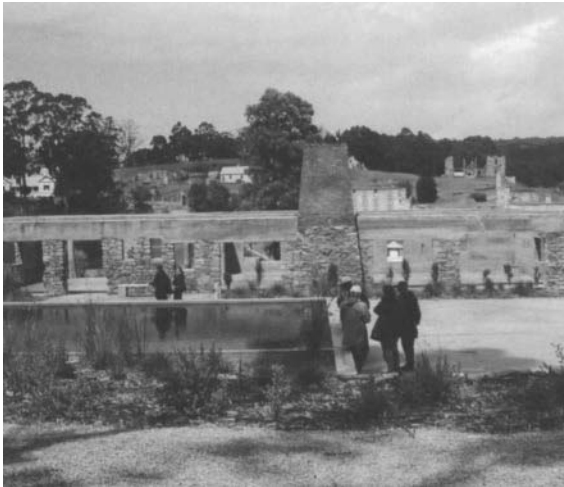
Port Arthur Memorial Garden. Demolition of the café was started shortly after the 1996 tragedy but was halted by court order. The structure remained in ruins until it was reconstructed as a memorial. The memorial, however, is not given prominence in the interpretation schemes of Port Arthur and serves primarily as a quiet testimony to the senseless killing of staff and visitors. Photo: Marta de la Torre
