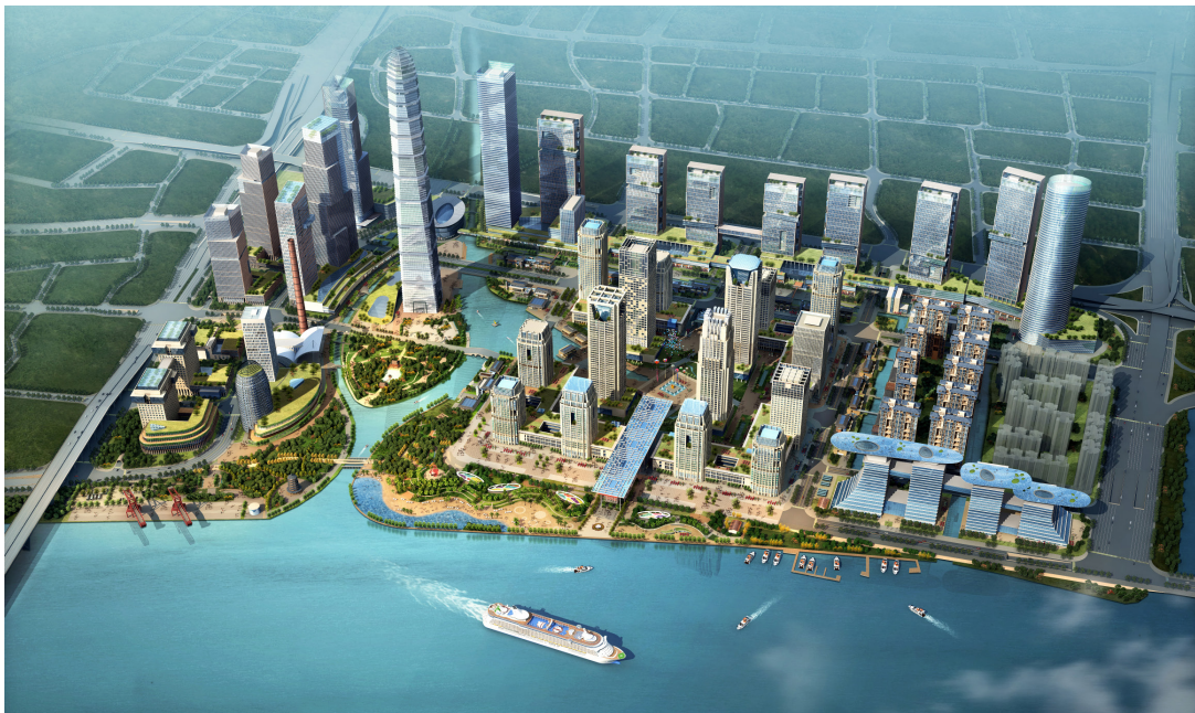
The Aerial View of Starting Area of Guangzhou International Financial City
