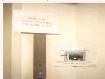
Restrictions imposed on employee elevator use to conserve electricity
