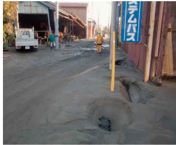
Sawmill affected by liquefaction in Katori City, Chiba Prefecture
