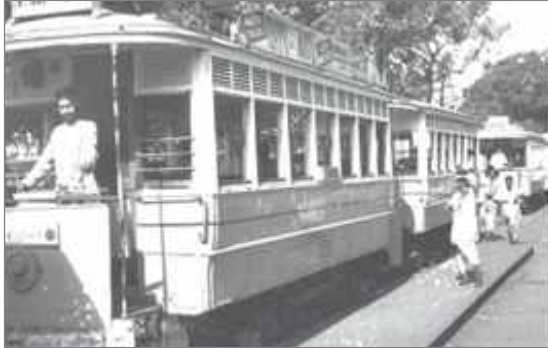
Before concretization Boarding/alighting stop for tram users
