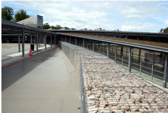
Figure 1. Besancon FC TGV (D.Zaluski). Additional thermal insulation delivered by its green roofs and the shape of the building itself.
