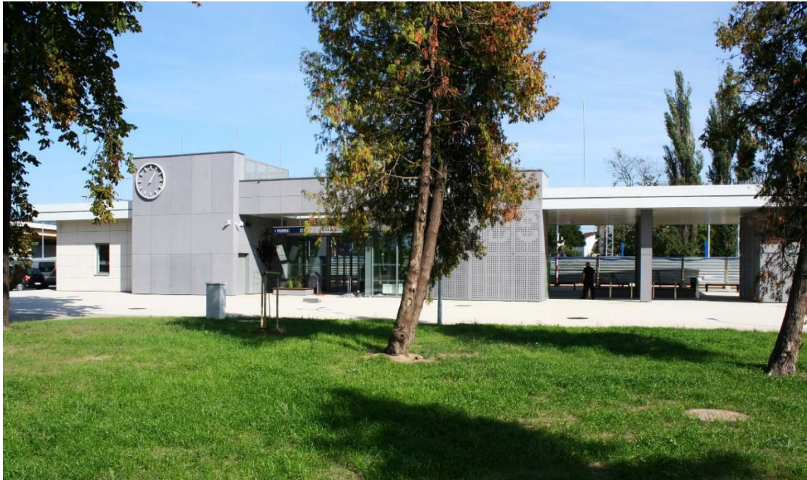
Figure 6. Innovative Railway Station in Mława (D.Załoski). A compositional dominant in a front view - a seven-meter-tall clock tower firmly identified with traditional station buildings. The maximum of existing trees have been maintained in Mława
