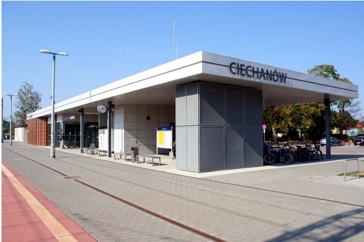
Figure 5. Innovative Railway Station in Ciechanów (D.Załoski). A seasonal waiting room shaded and well protected from the rain by a large field of the extended roof. Also a place for bicycle racks, vending machines, storage lockers and ATMs
