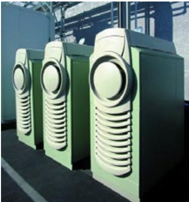
Figure 2: Micro-turbine installation
