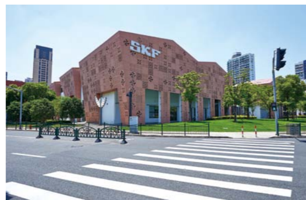
SKF's green building
