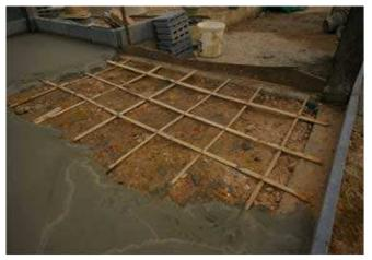
Fig7: Bamboo Reinforcement
