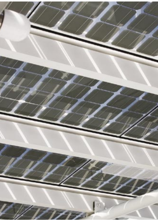
A 13.1kW array of building integrated photovoltaic panels complements other energy-saving features such as high-efficiency water source heat pumps, microturbines and occupancy sensors.
