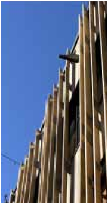
Figure 05: Sidwell Friends Facade Detail (AIA Cote Top Ten, 2007)
