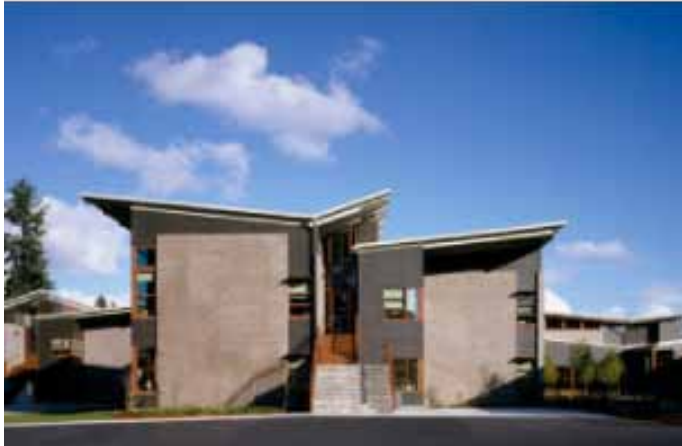
Figure 08: West Elevation View of Ben Franklin Elementary School
