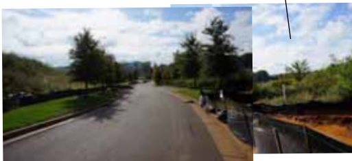
Figure 24: Photos from the site
