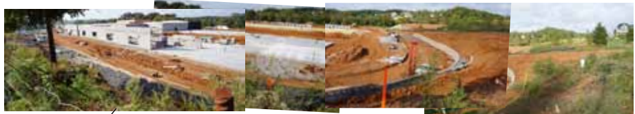
Figure 23: Photos from the site
