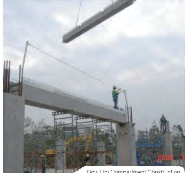
Dow Dry Compartment Construction
