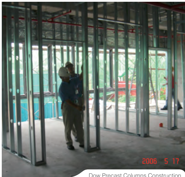
Dow Precast Columns Construction
