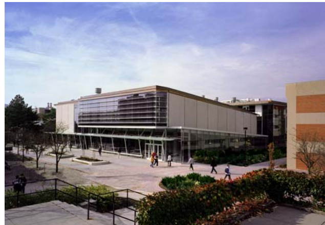
Figure 9. York University Computer Science Building
