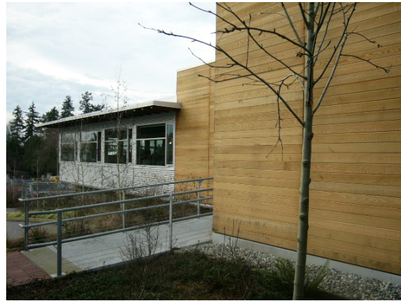
Figure 6. White Rock Operations Building
