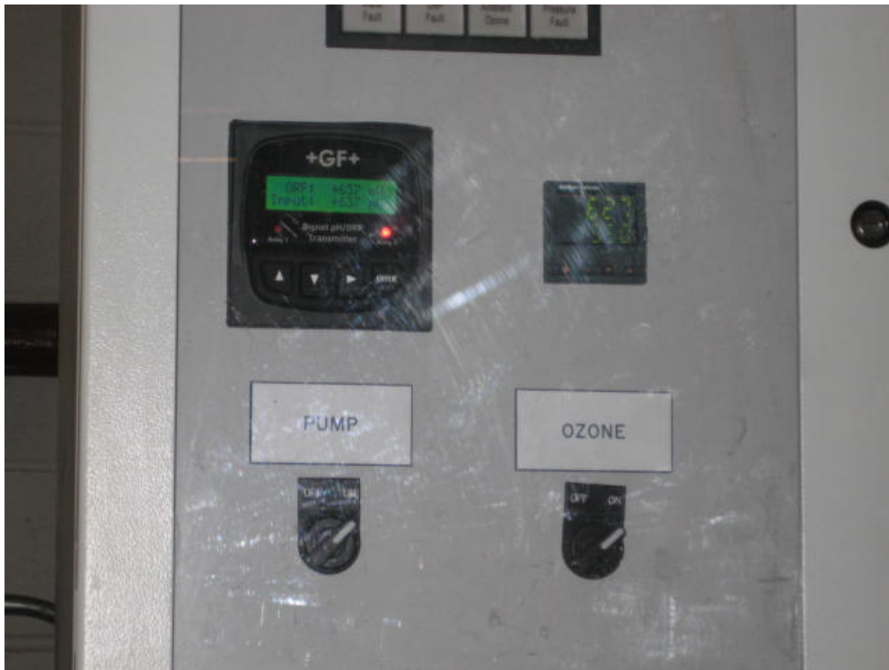
Figure 2-40 Controls for pumping and ozonation
