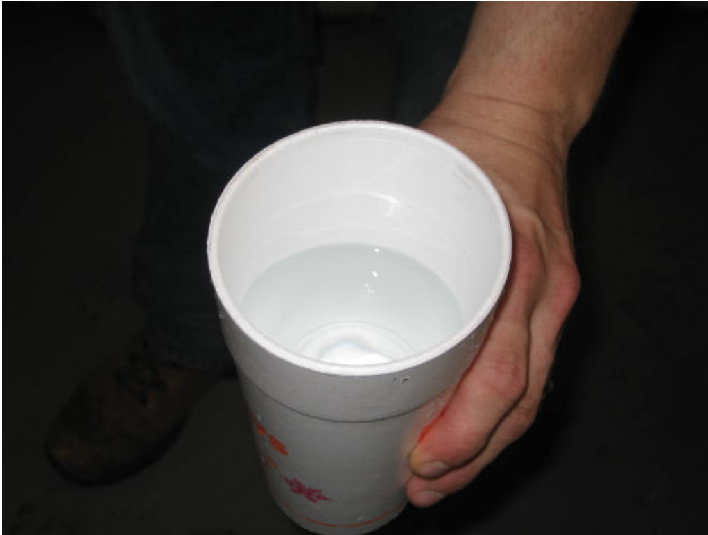
Figure 2-41 Finished water from onsite blackwater reuse plant
