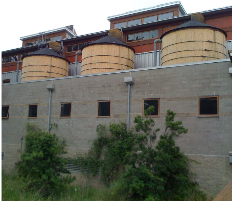
Figure 2-15 Merrill Center roof catchment photo
