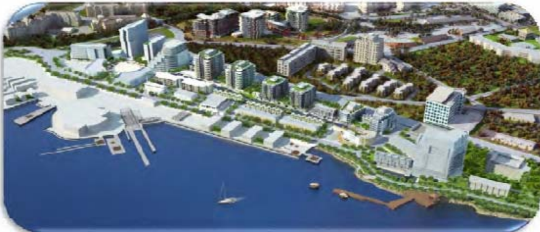
Figure 4-5 Rendered view of Dockside Green, Victoria, BC, Canada Source: Used with permission from (Dockside Green, 2009)
