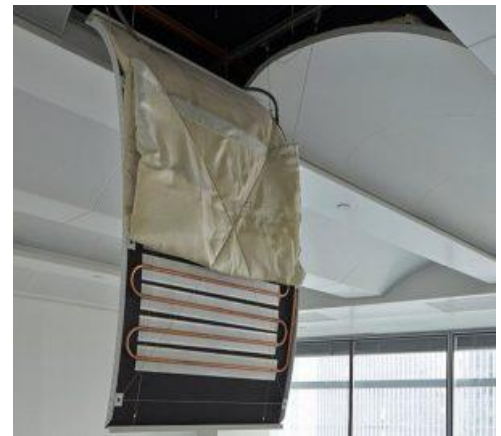
Radiant Cooling System. Photo Courtesy of AGU.
