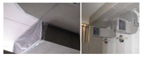
**Figure 3 :** New elementary school of Romarzollo (Arco-Italy)- Covered HVAC ducts in conformance with the IAQ PIndoor Air Quality Management Plan during Construction.
