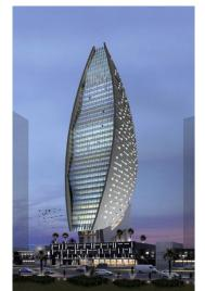
objective not by the normal height differentiator, but by its form. The distinctive design comprises two identical double curved pixelated shells which are rotated and cantilevered over the podium. The rear elevation is a continuous vertical curve punctuated by balconies while the front elevation is made up of seven zones of rotated glass.
